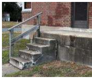
36" tall landing missing guardrail
